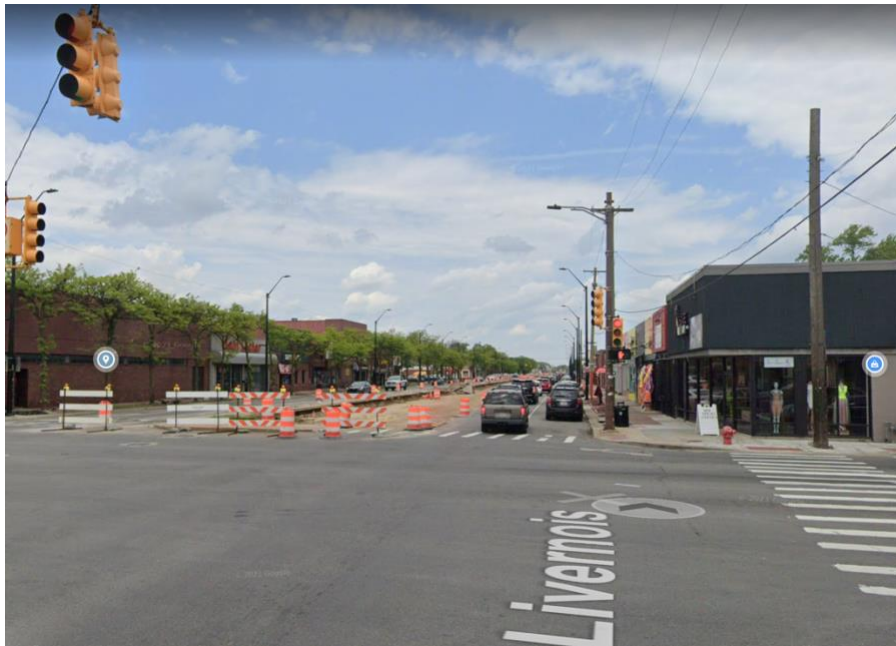
Figure 1: Former state of Livernois Avenue
