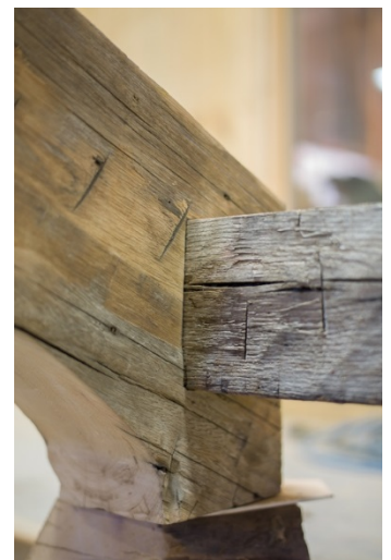
Figure 3: Reclaimed Timber Frame
