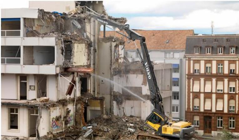
Figure 2.11. High Reach Excavator with a boom reach of 21-32 meters.
