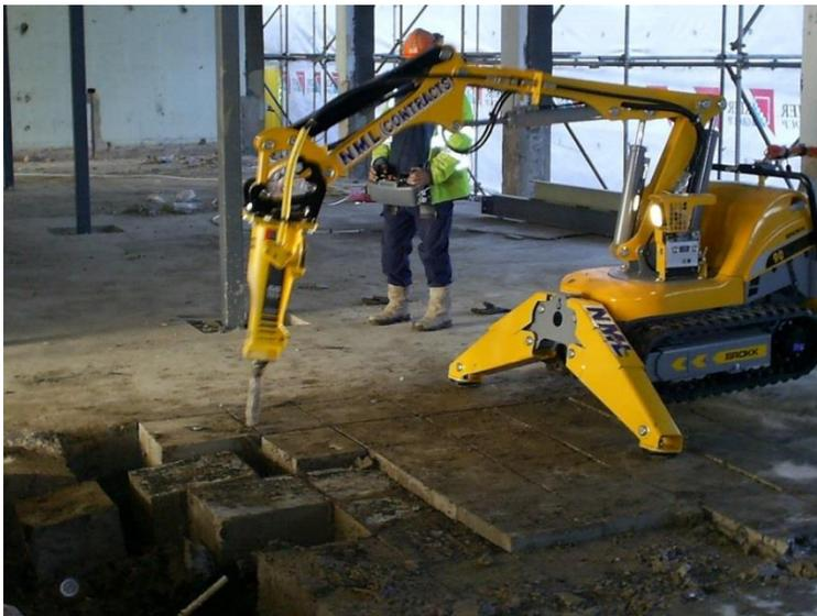
Figure 2.18. Robotic machine used for selective demolition of concrete flooring with a concrete cutter.
