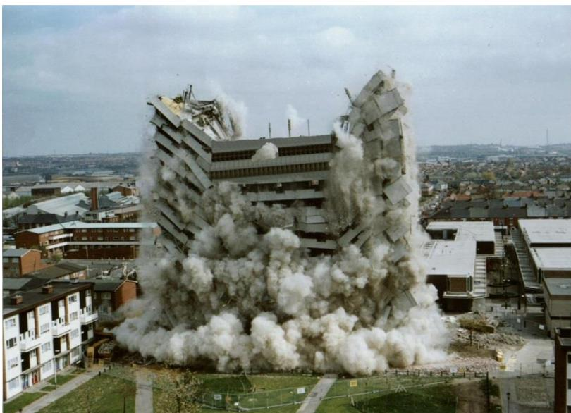
Figure. 2.20. Controlled implosion of a high-rise building.
