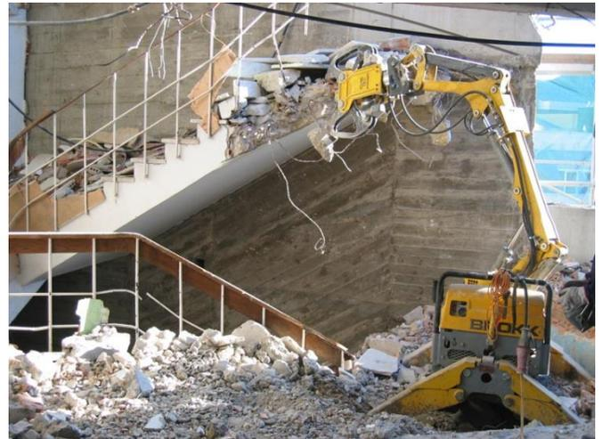
Figure 2.6. Robotic concrete cracker being controlled by a joystick.
