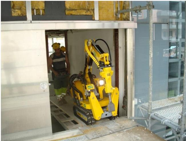
Figure 2.5. Robotic concrete splitter being controlled by a joystick. A lot of different attachments can be used with these machines
