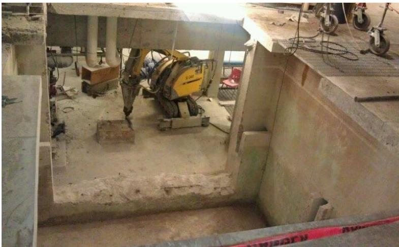
Figure 2.17. Robotic excavator breaking concrete in the basement floor.
