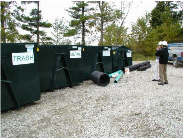
Figure 2.22. Using containers for sorting material on site
