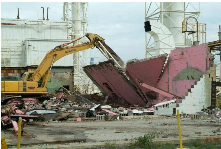
Figure 2.15. Crawler excavator pulling down walls.
