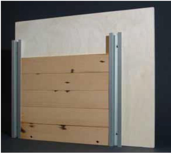
Figure. 2.42. Siding attached with double stick tape.
