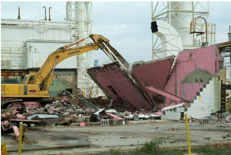
Figure 2.15. Crawler excavator pulling down walls.
