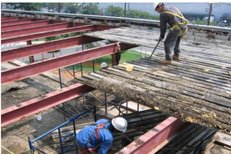
Figure 2.19. Removing flooring sheets by simple hand tools is an example of selective demolition
