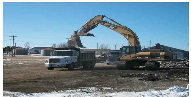
(Figure 8. Crawler excavator loading debris into trucks used for hauling away the material to landfill
