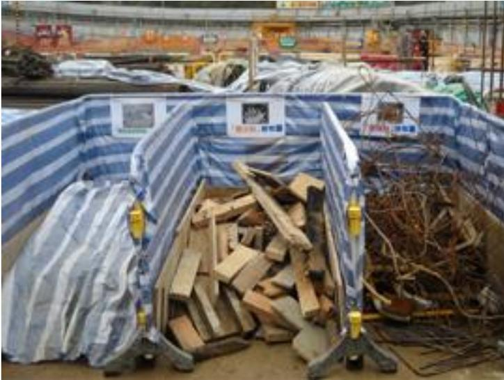
Figure 2.21. Sorting material by type results in efficient flow of operations on site. The pictures show different ways of creating stacks for material.
