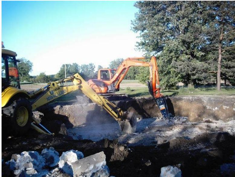
Figure 2.16. Excavators digging out foundation concrete. The wheel excavator is using the bucket to remove the material where the crawler excavator is using the concrete cracker attachment to break the concrete
