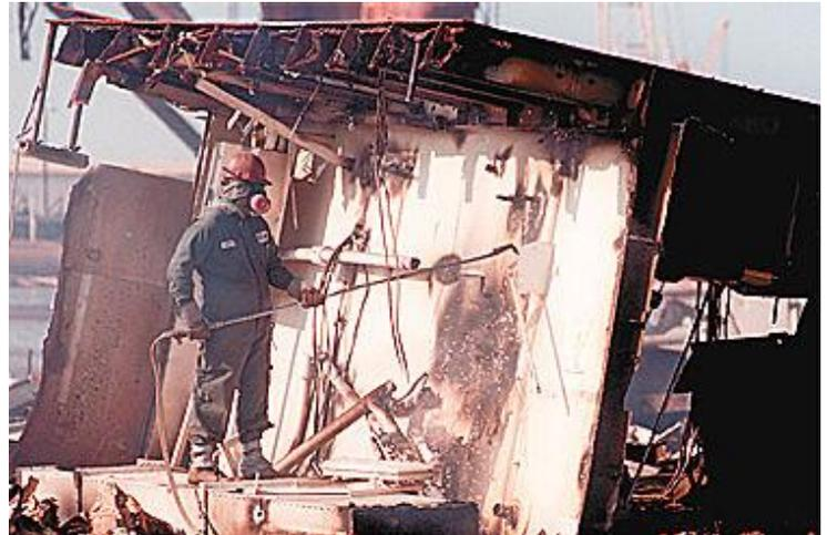
Figure 2.10. Steel cutting torches are used for selective demolition of steel structures
